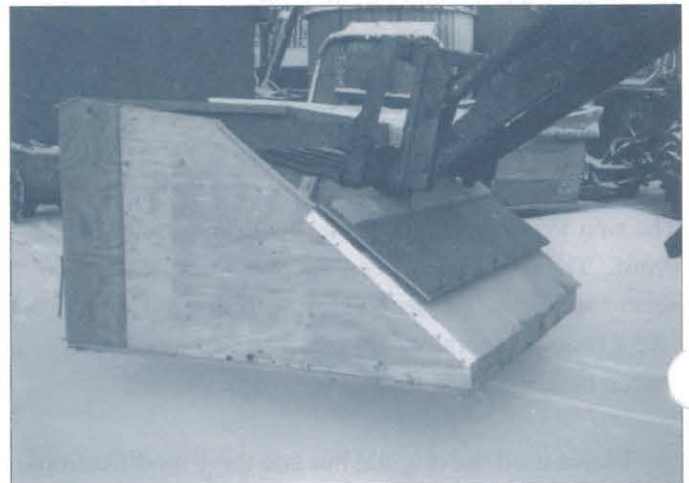
The hut can be lifted and moved by its oak roof beam.
