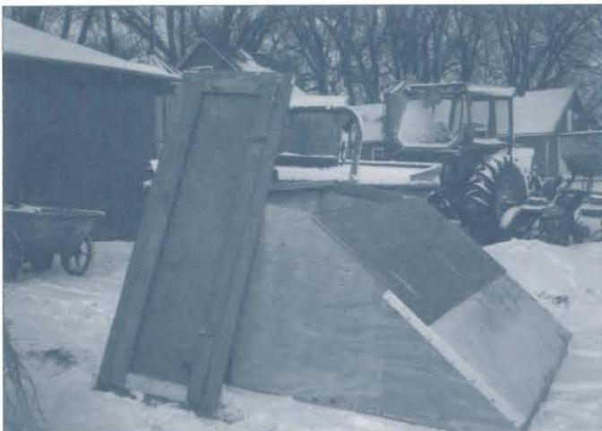
Roof lid showing pins that hold rear vent door closed.
