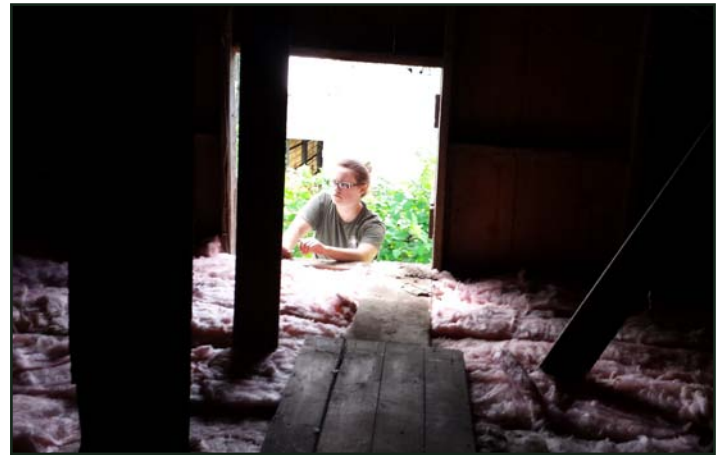
Green Iowa Americorps insulate the ceiling of the chicken coop.
