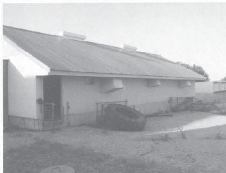
The view from the outside of the confinement farrowing building.
