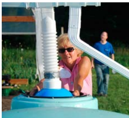
Linda Naeve demonstrates how rainwater collects in a large tank and is then diverted to a gutter once the tank is full.
