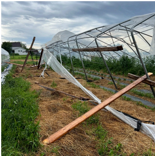
Photo depicts recent wind damage at Sweet Season Farm
